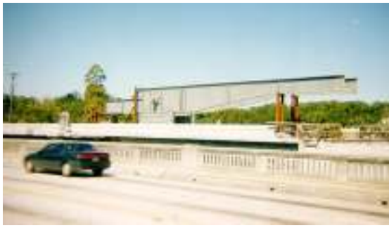
Figure 1 Trunnion-Hub-Girder (THG) assembly.
